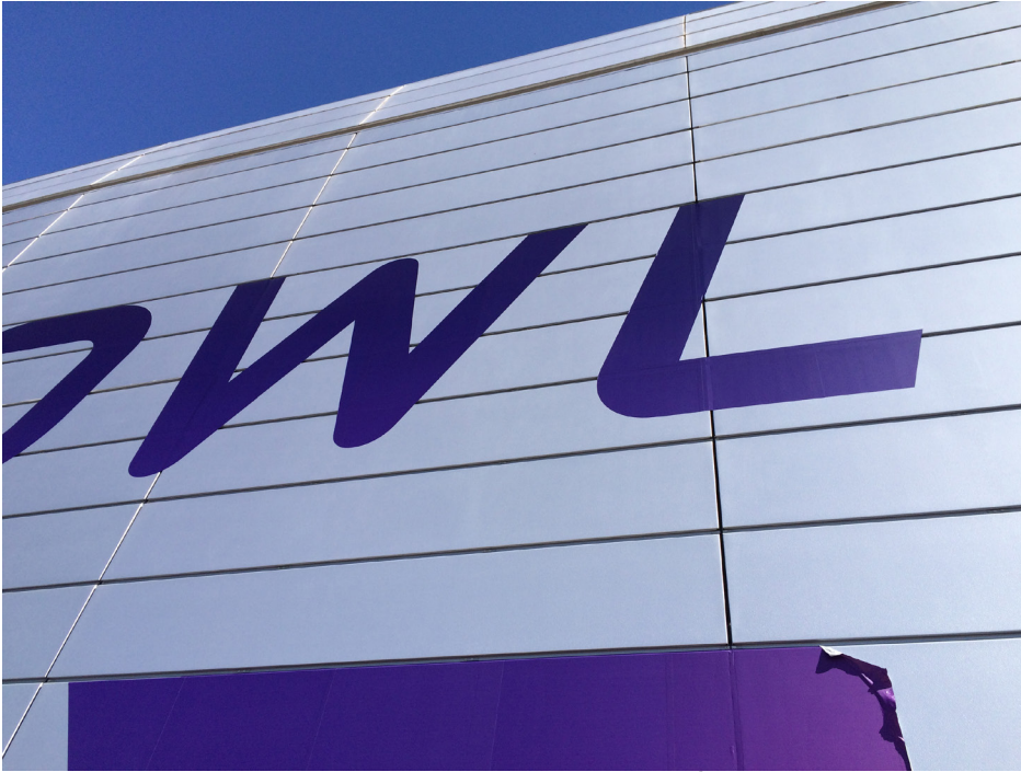
Figure 3. Start point of removal from upper left corner of a warm graphic
